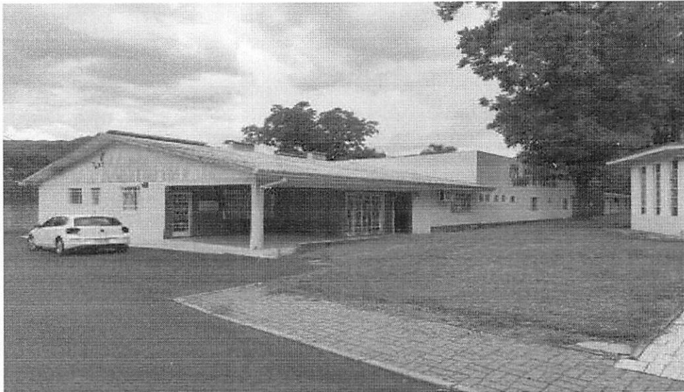
Fachada do bloco principal
