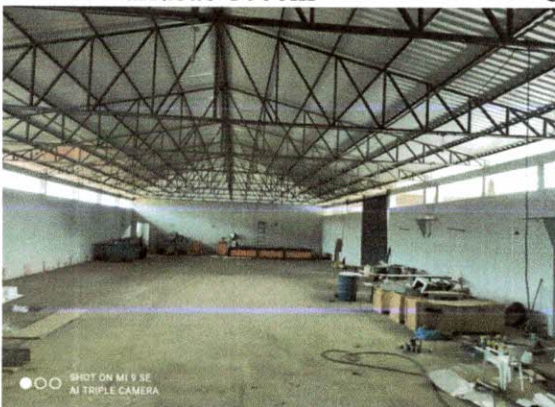
Interior Barracão 600m 2
