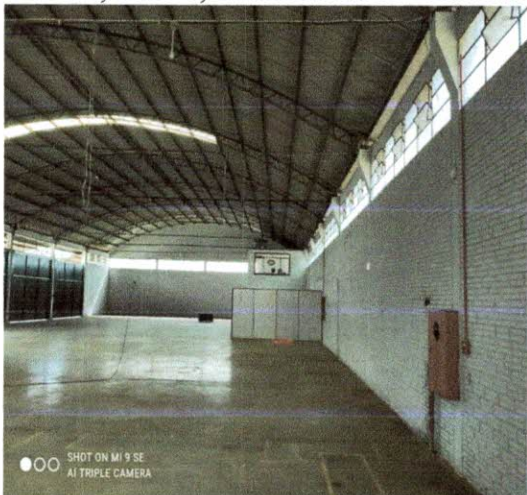
Interior Barracão 1000m 2
