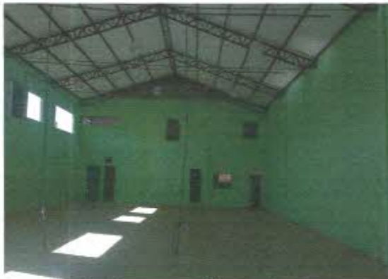
Interior do Barracão e bw, salas
